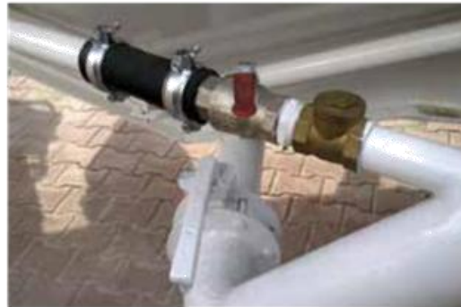
5- The red valve (jet valve) should be \frac{1}{2} open. The white valve is for discharging, it must be full open like this sample.
